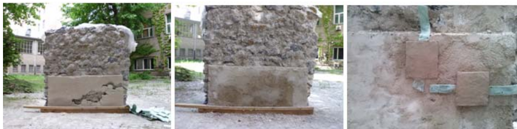
Fig. 2. Lacunae in the arriccio of the testing masonry. The plaster was applied only in the lower portion of the wall (a). After the mapping, the lacunae were covered with a thin layer of plaster sustained by a tissue (b). Detachment of the finishing layer (c).
