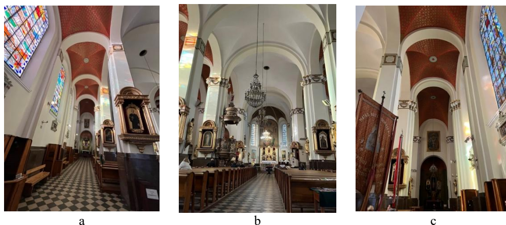
Fig. 15. View of the vault: a) in the left-side aisle; b) in the main nave; c) in the right-side aisle
