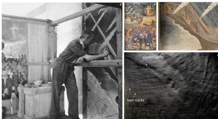
Fig. 14. Mural P3 at Alcântara: (a) historical photograph taken during its pictorial execution in 1945; (b) corresponding detail recorded in 2021 under visible light; (c) the same area recorded under visible raking light, highlighting plaster joints, surface irregularities, and tool marks, Image sources: ANSA-F-246, CEDANSA - NOVA FCSH / © Estate of José de Almada Negreiros and Manuel Ribeiro, 2021.
