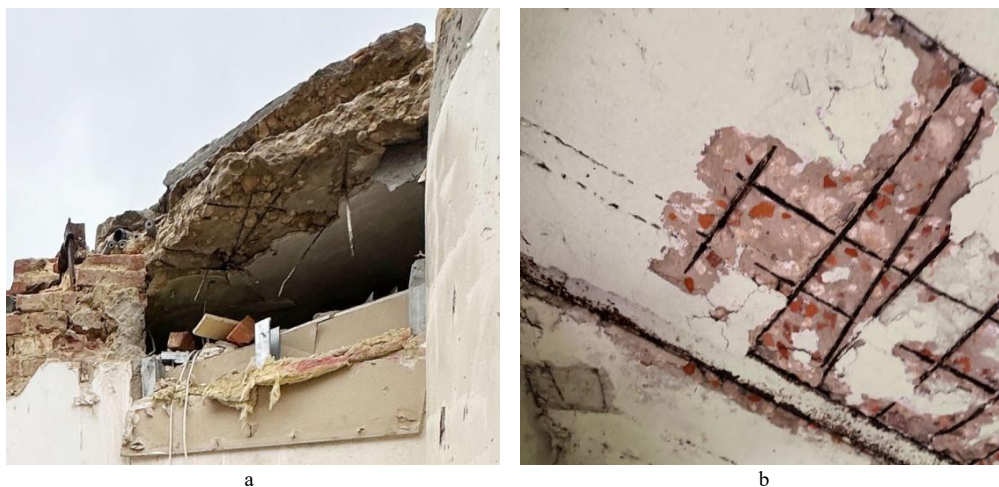
Fig. 6. Early reinforced concrete at 44 Konovaltsia Street: view of the third floor (a) an fragment of the ceiling (b), documented on 28 January, 2025 (photo: Ihor Bokalo)
