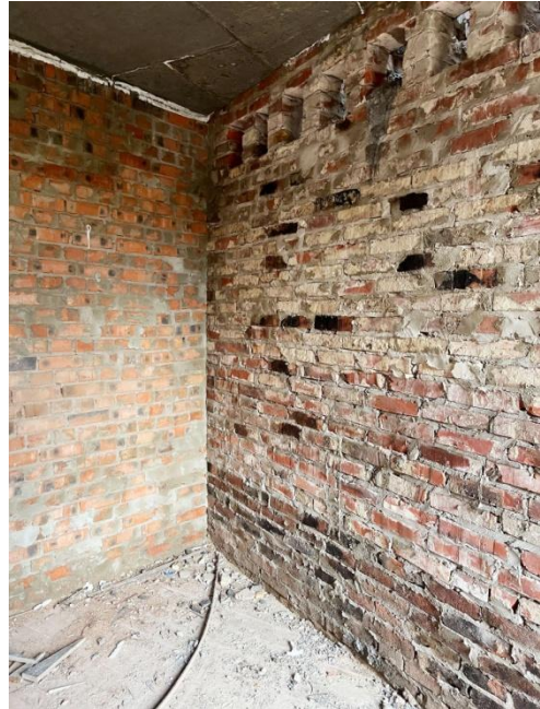
Fig. 19. Wall masonry composed of contemporary and historic bricks at 64 Stryiska Street, documented on 20 October 2023 (photo: Ihor Bokalo)
