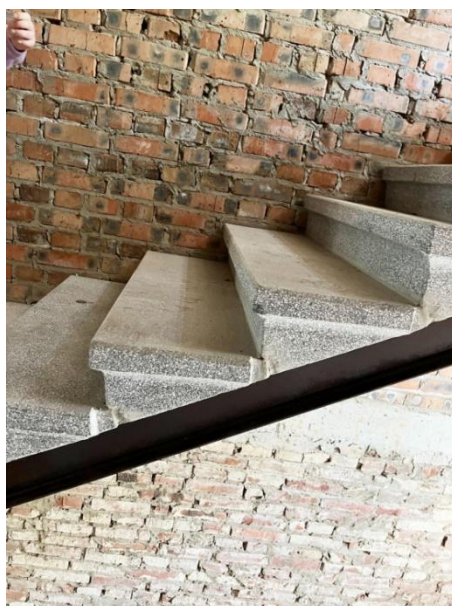
Fig. 21. Reconstructed contemporary prefabricated reinforced concrete stair treads installed on steel stringers in Building No. 64 on Stryiska Street during the reconstruction process, documented on 29 April 2024(photo: Ihor Bokalo)
