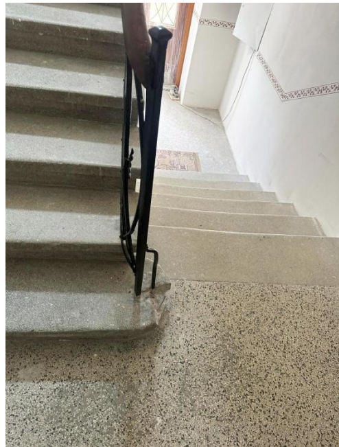
Fig. 16. Historic stairs finished in terrazzo in Building No. 68 on Stryiska Street during the restoration works, documented on 11 June 2025 (photo: Ihor Bokalo)
