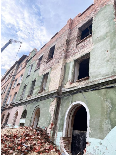
Fig. 18. Rear façade of Building No. 64 on Stryiska Street during the restoration process, documented on 20 October 2023 (photo: Ihor Bokalo)
