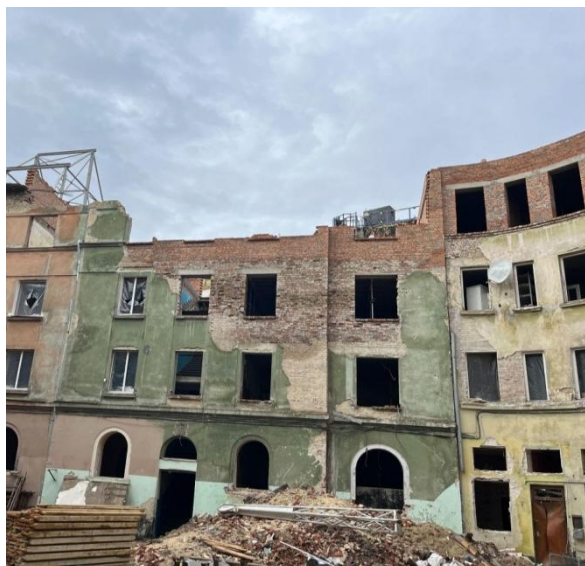
Fig. 1. 64 Stryiska Street: view of the facade from the inner courtyard documented on 20 October 2023 (photo: Ihor Bokalo)
