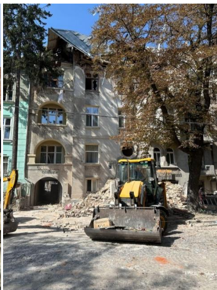
Fig. 2. Main façade of 44 Konovaltsia Street shortly after the missile attack, documented on 4 September 2024 (photo: Mariana Kaplinska)
