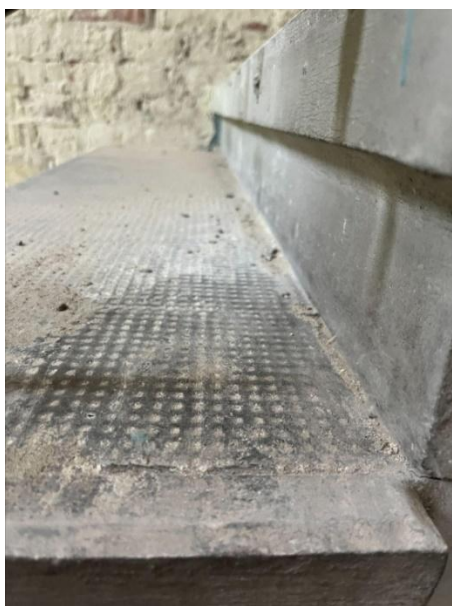
Fig. 20. Historic prefabricated reinforced concrete stair treads with factory-applied bush-hammered surfaces, intended as a base for the terrazzo finish, in Building No. 68 on Stryiska Street, documented on 19 March 2025 (photo: Ihor Bokalo)
