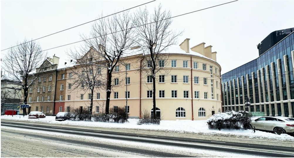
Fig. 22. View of the restored residential complex on Stryiska Street from the north, documented on 9 January 2025 (photo: Mariana Kaplinska)
