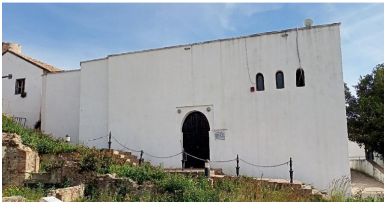
Fig. 20. The south façade
