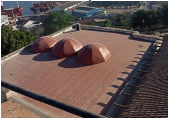
Fig. 14. The roof's current state
