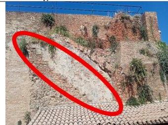
Fig. 11. Traces of stairs
