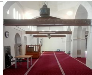
Fig. 7. Position of wooden tie beams
