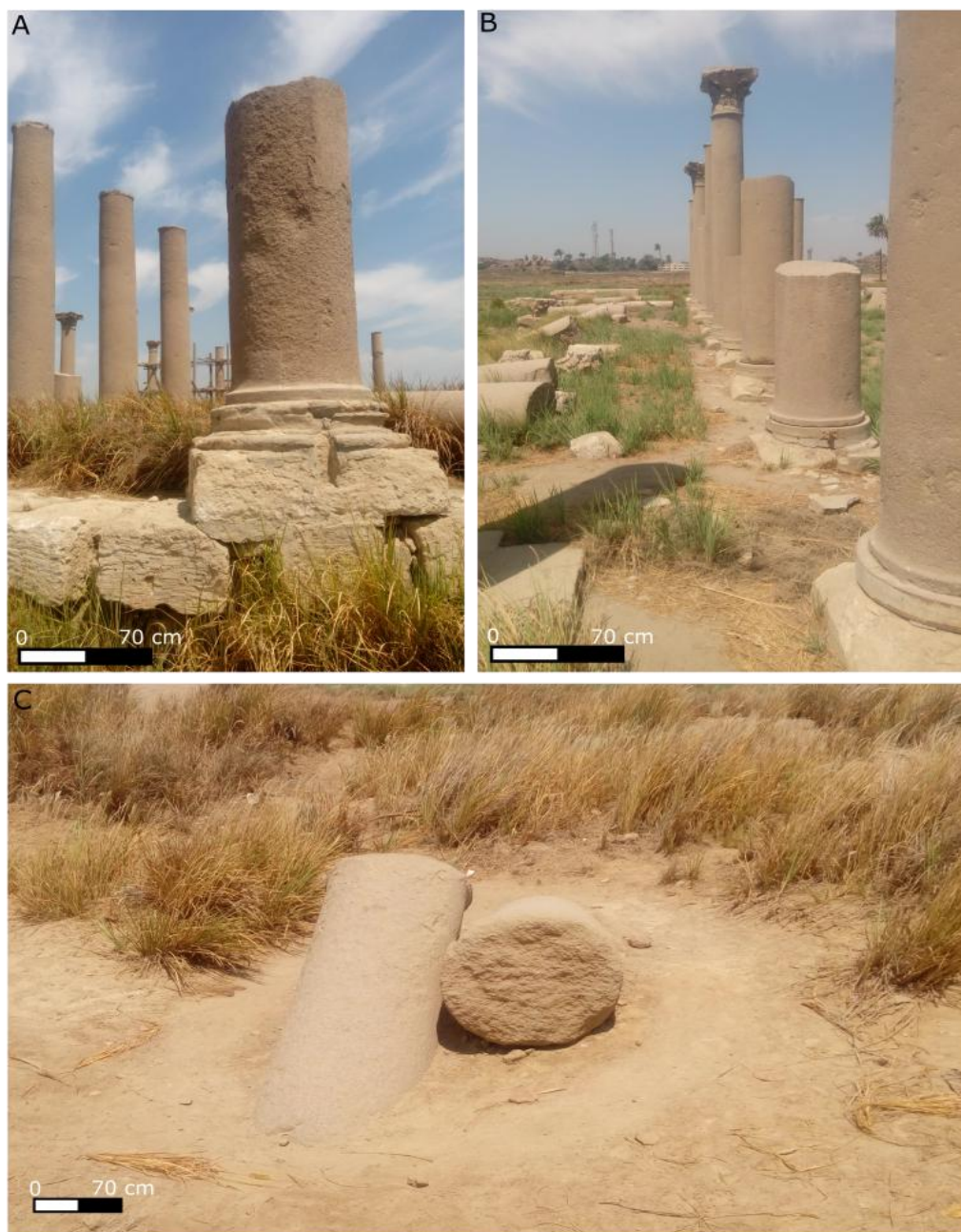
Fig. 1. (A-C) the columns exhibit various types of damage, including surface erosion from weathering, mechanical breakage and fragmentation of shafts and drums, biological deterioration from surrounding vegetation, structural instability leading to displacement and toppling, and potential foundation issues causing uneven settling and misalignment
