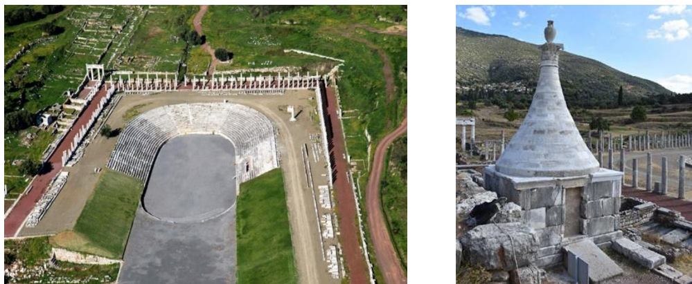
Fig. 1. The Stadium and the Gymnasium of Ancient Messene after restoration and Funerary monument K3 after its restoration [13] ( https://pacf.gr/etaireia-messiniakon-archaiologikon-spoudon-2/ )
