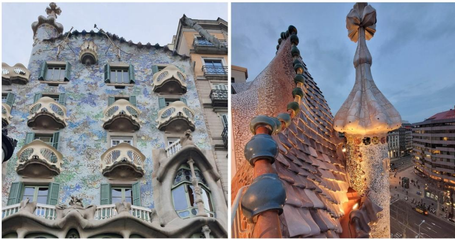
Fig. 1. Casa Batlló's organic forms
