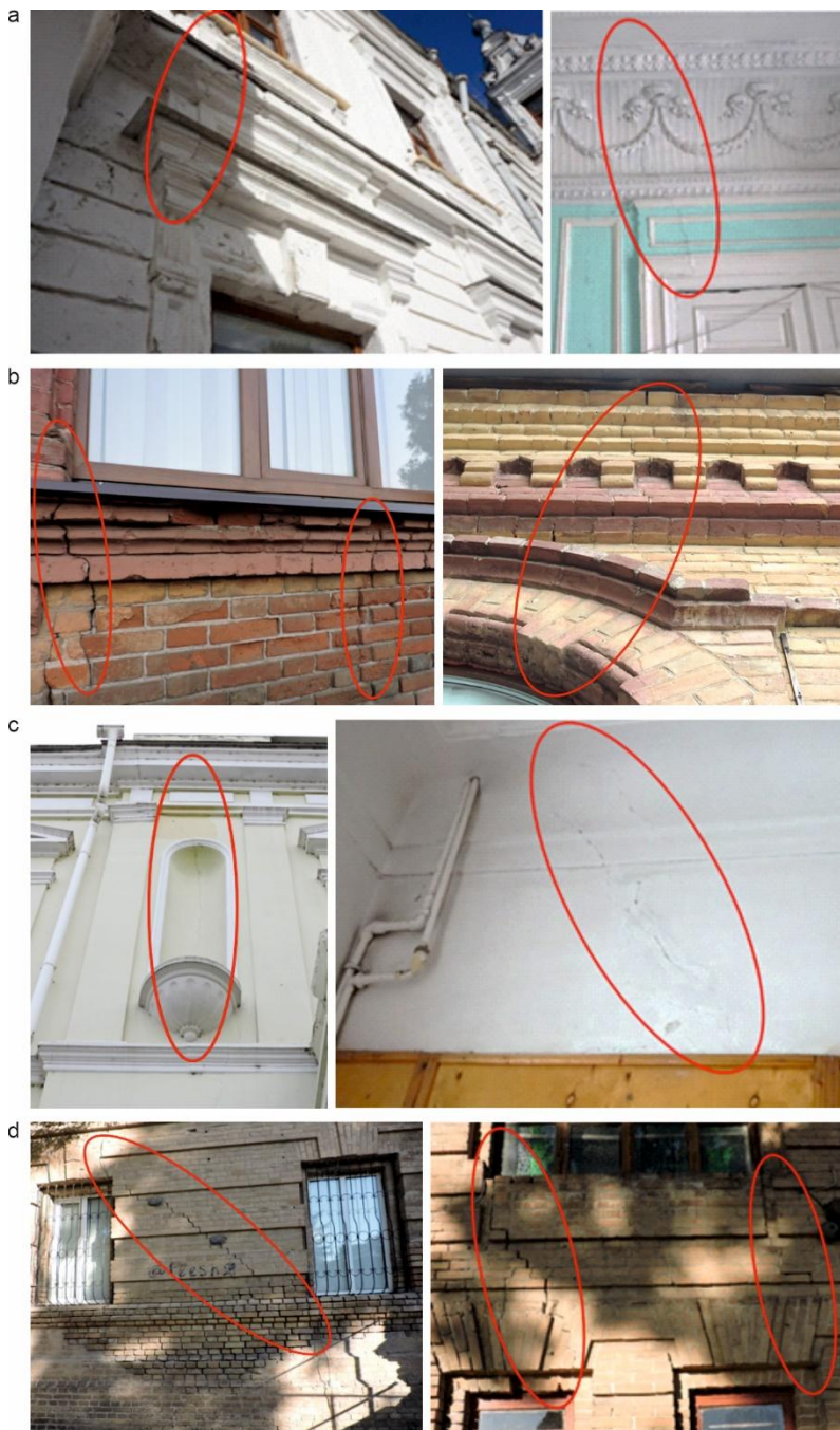
Fig. 2. Examples of historical buildings' cracked walls: a – Andrushivka Lyceum No. 1 with a primary school (Zhytomyr region); b) Balta Oles Gonchar Lyceum No. 1 (Odesa region); c) Izmail Lyceum No. 1 (Odesa region); d) Izmail Gymnasium No. 2 (Odesa region).
