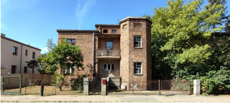
Fig. 2. The villa, current view from Grochowska Street, current state.
