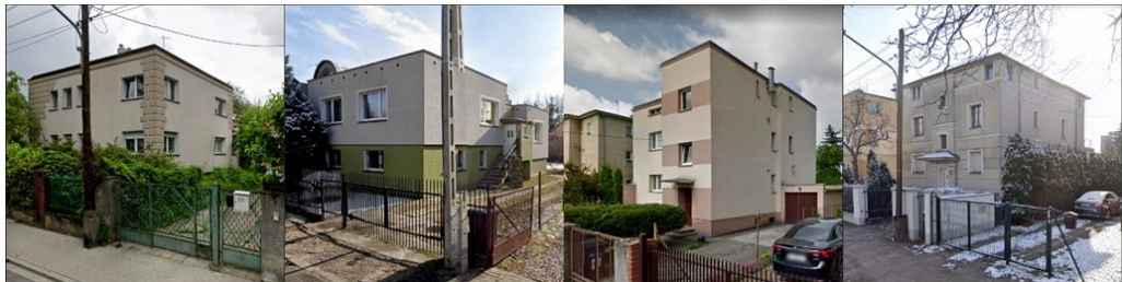
Fig. 9. The study includes a selection of negative examples of modernization interventions carried out on modernist buildings located in the ‘Abyssinia’ district. These cases were analyzed to highlight the consequences of inappropriate renovation practices, including the loss of original architectural features, the use of incongruous materials, and the introduction of stylistically inconsistent elements. By documenting these unsuccessful transformations, the research aims to identify common errors and oversights that compromise the historical and aesthetic value of early 20 th -century modernist architecture. These examples serve as a critical reference point in shaping responsible design strategies for future conservation and adaptation projects.
