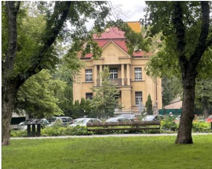
Fig. 9. Jadwiga Villa, present condition
