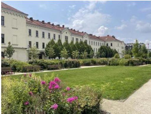
Fig. 4. Provincial Public Library, present condition
