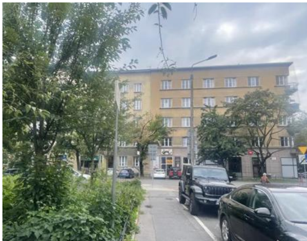
Fig. 14. Buildings in the immediate vicinity. Present condition
