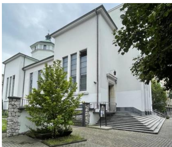
Fig. 12. St. Stephen's Church, present condition
