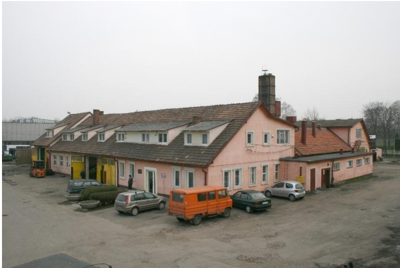
Fig. 3. The building of the former camp slaughterhouse used by the bus depot – before the investment (photo: "Kozień Architekci" Archive)
