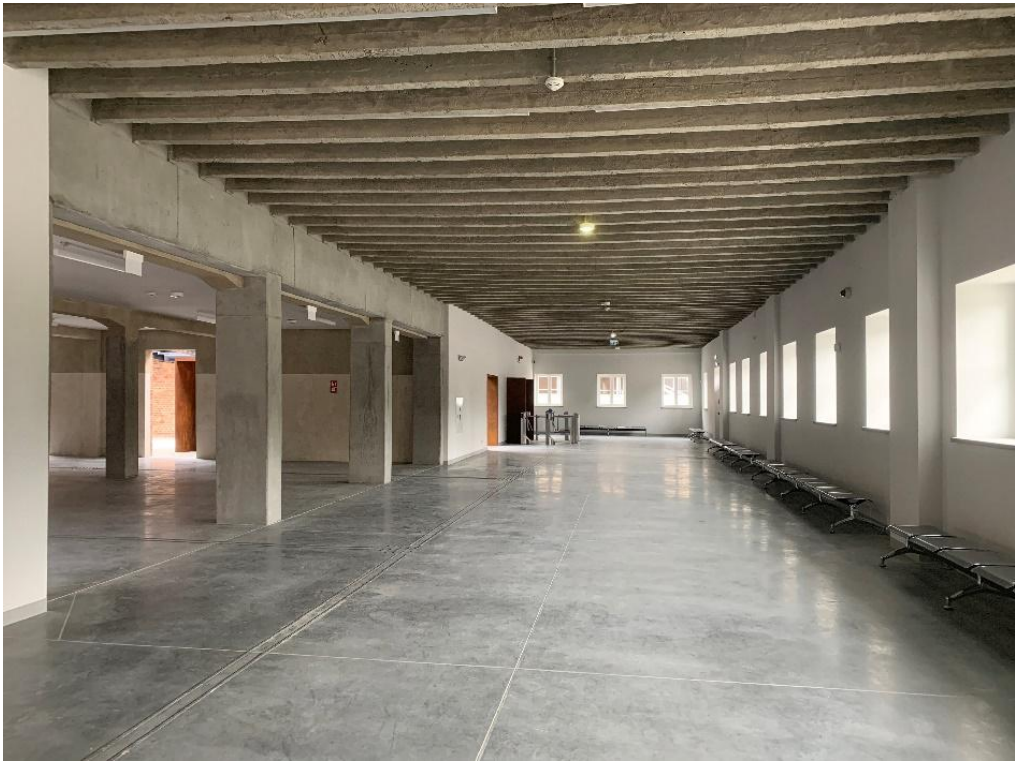
Fig. 11. Adaptation by “Kozień Architekci” of the hall with original ribbed concrete ceiling in the former camp slaughterhouse – now the Visitors’ Center of the Auschwitz-Birkenau State Museum in Oświęcim (photo: “Kozień Architekci” Archive)
