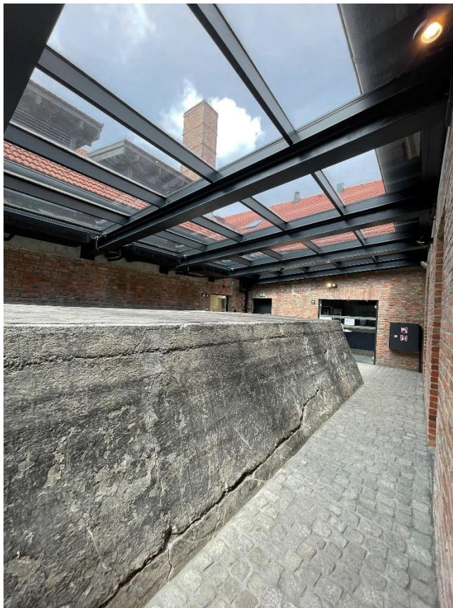
Fig. 6. Adaptation by “Kozień Architekci” of the courtyard of the former camp slaughterhouse and historic bunker – now the Visitors’ Center of the Auschwitz-Birkenau State Museum in Oświęcim (photo: “Kozień Architekci” Archive)
