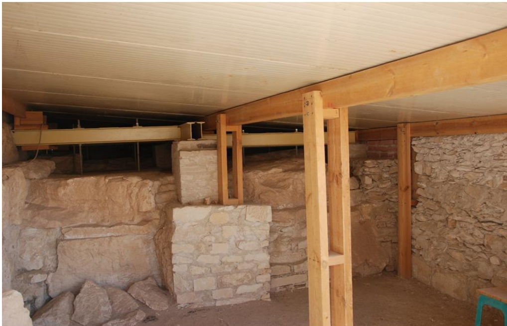
Fig. 5. Strengthening and roofing the vestibule of the Hathor Chapel.
