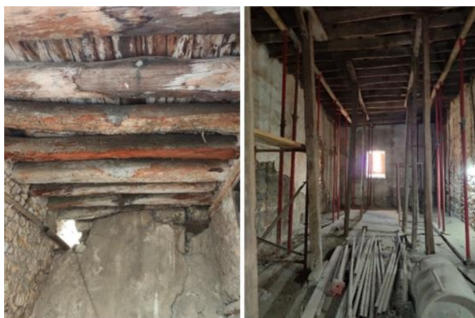
Fig. 2. Basement below the museum
