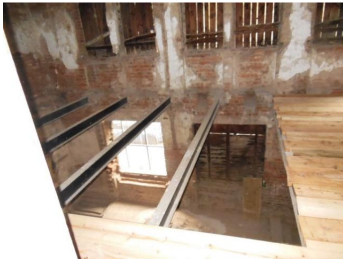
Fig. 2. New steel I-beams, CPNMBiH, 2016
