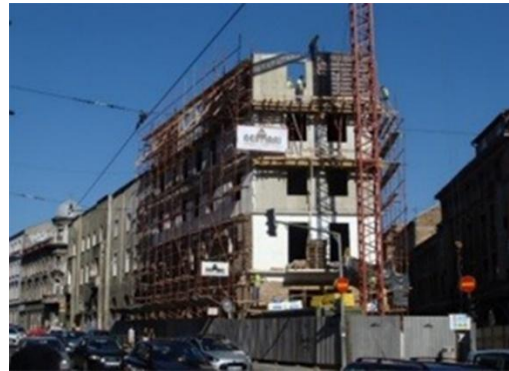
Fig. 14. Hotel Zagreb with the reconstruction in progress in 2014
