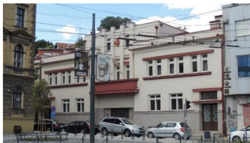
Fig. 6. Facade after the completion of the reconstruction (2023)
