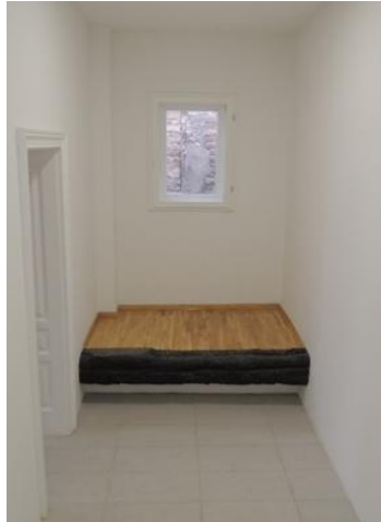
Fig. 3. Bosnian Red Cross Society building in Sarajevo: preserved original carbonized wooden beam integrated into a new interior; actual state in 2016
