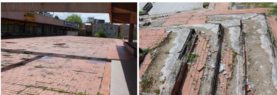
Fig. 18. Skenderija cultural and sports center, destroyed paving of the open space due to a lack of maintenance (2021)
