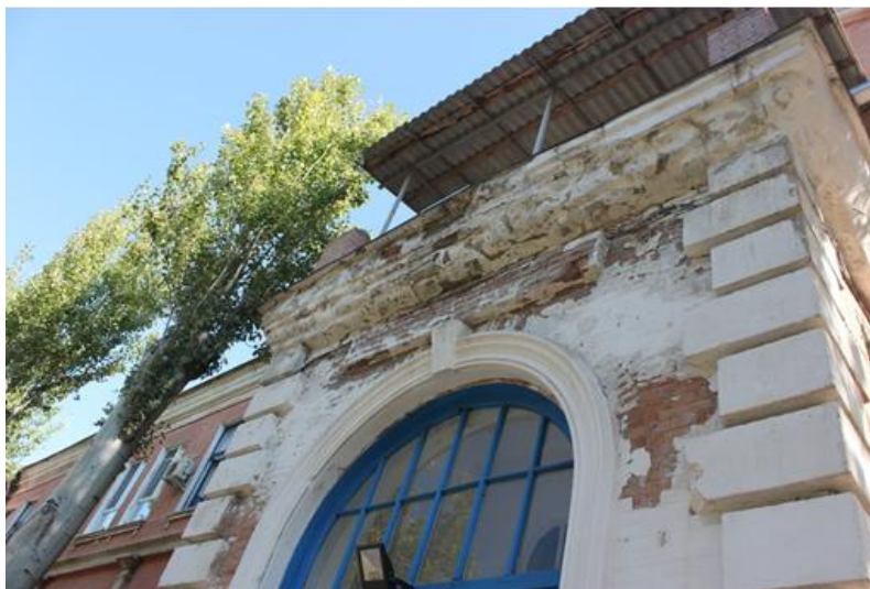
Fig. 4. Fragment of the external walls.
