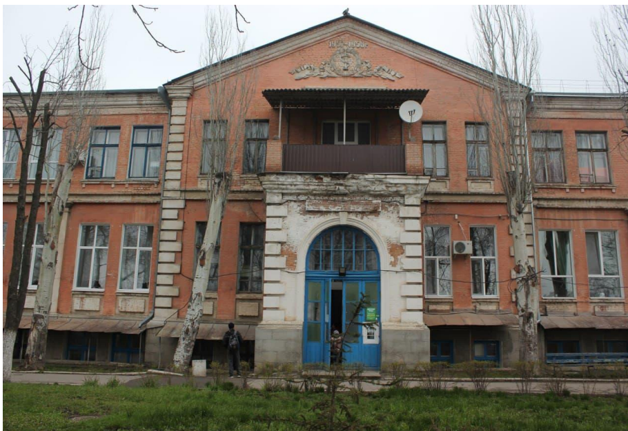
Fig. 1. The main facade of the medical building No. 2 (state before restoration).
