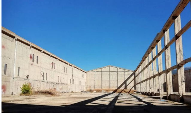
Fig. 7. Photograph of the building under study
