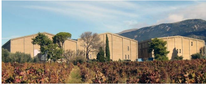
Fig. 6. Photograph of three buildings next to the historic ones to facilitate the winery
