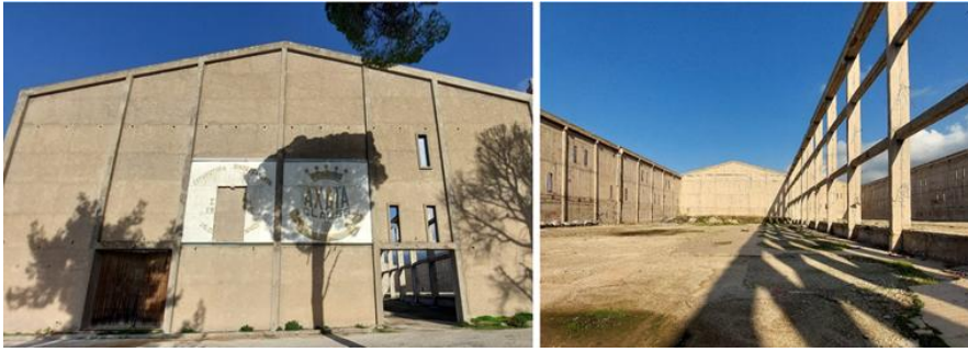
Fig. 24. Front and interior views of the building under study
