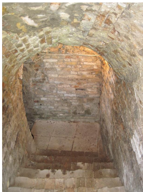
Fig. 5. Infiltration of atmospheric precipitation due to violation of waterproofing (underground structure No. 2).
