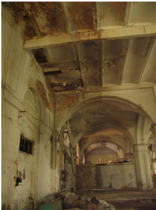
Fig. 5. Emergency condition of the vaults before restoration. From the stocks of the Ukrrestavratsiia corporation
