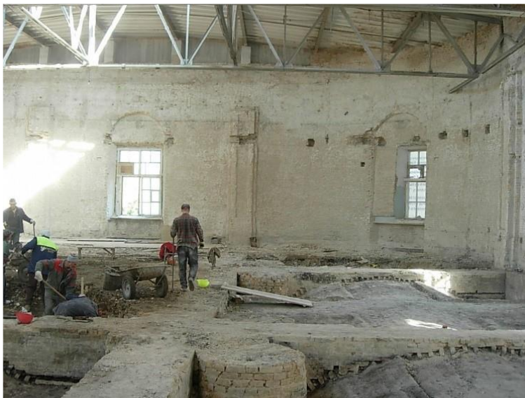
Fig. 7. Strengthening the foundations of the Mystetskyi Arsenal. From the stocks of the Ukrrestavratsiia corporation
