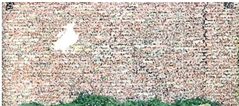
Fig. 5. Visualization of a LiDAR scan of a wall with a structural deficit
