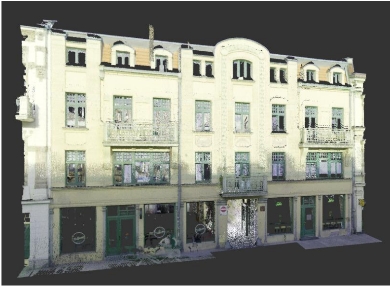
Fig. 4. The point cloud of the front elevation of the tenement house at 41 Piotrkowska Street in Lodz
