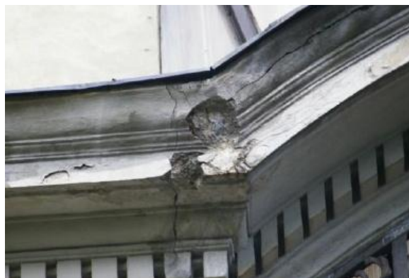
Fig. 4. Visible crack on the roof (Photo by “Marciniak & Witasiak Architekci”)
