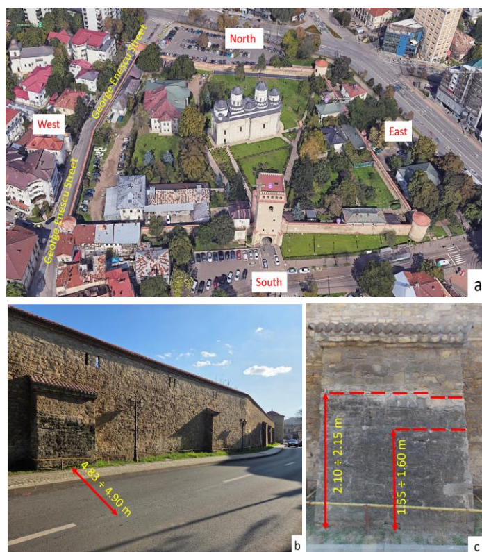
Fig. 1. Site context and geometry of the investigated wall section at Golia Monastery (Iași, Romania): (a) aerial view of the Golia Monastery ensemble, showing the orientation of the west wall parallel to George Enescu Street and the relative position of cardinal directions (North–South–East–West) (source: Google Earth); (b) street-level view of the western wall and buttresses, with the roadway axis located approximately 4.83–4.90m from the wall base; (c) detail of the investigated buttress, showing the black-crust band (~1.55–1.60m) and the substrate reference band (~2.10–2.15m) used for comparative pXRF measurements
