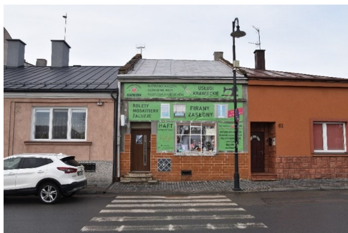
Fig. 13. View of a section of the western frontage of the market and the façade of the single-story house Rynek 60, which is almost entirely covered with advertising banners. Existing condition
