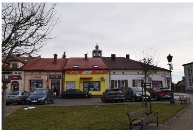
Fig. 11. View of a section of the eastern frontage of the market square and the façade of the pharmacy building (Rynek 31) in a color negatively distinguished from the neighboring buildings. Existing condition
