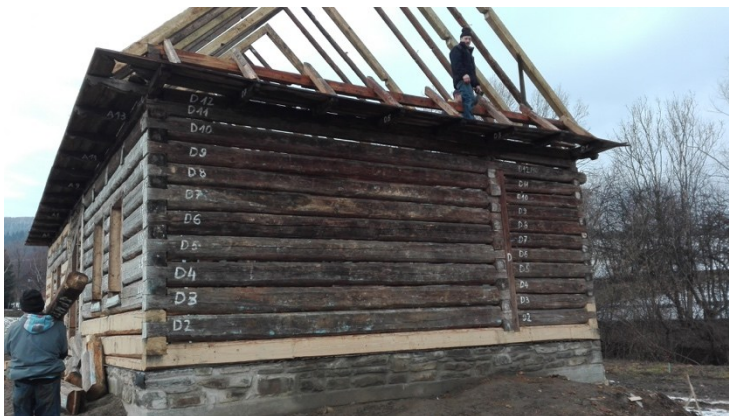
Fig. 2. Installation of marked construction elements in a new location (photo author)
