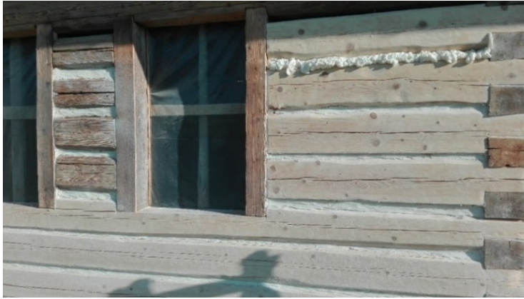
Fig. 3. Different phases of the process of sealing logs on one of the walls of the building (photo author)
