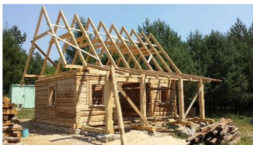
Fig. 7. House no. 3 under construction
