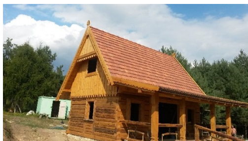
Fig. 8. House no. 3 in open shell state
