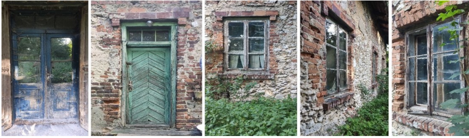
Fig. 6. Window and door woodwork, selected examples, 23/08/2022;
