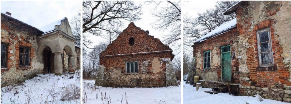
Fig. 3. Contemporary condition of the manor house - 22/02/2022, from the left: front elevation (west), north elevation, kitchen annex view; own photographs
