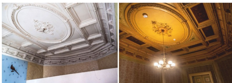
Fig. 9. Interiors of the Hilary Majewski Tenement House, elimination of secondary room divisions, and renovation of rich ceiling decorations. On the left, before revitalization in 2016; on the right, after the investment in 2022 (Photo by Stefan Brajter)
