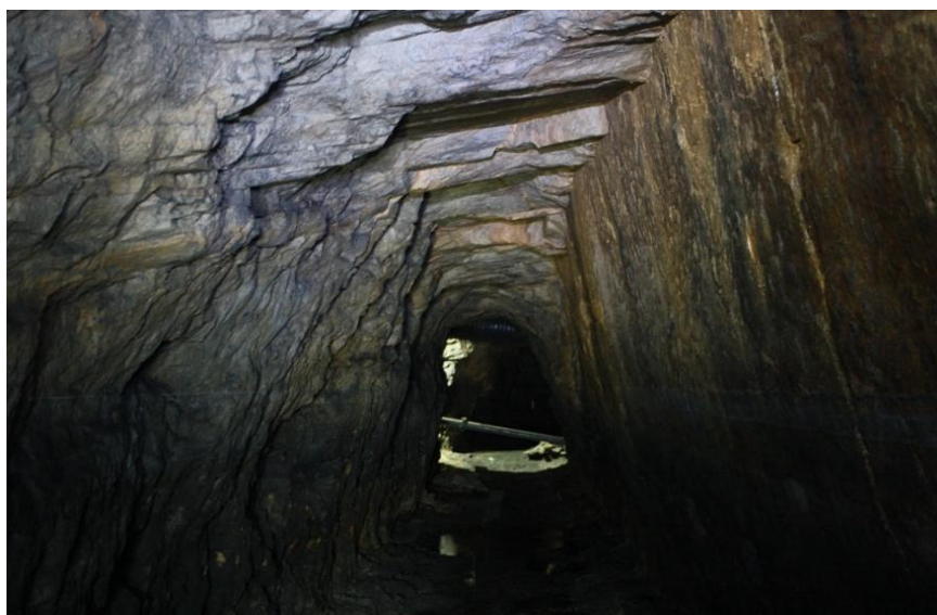
Fig. 9. Adit from link walkway 'B' (0m) to 86m wrought in sandstone (view towards the sub-pit). Width of corridor 160cm
