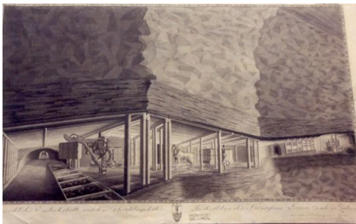
Fig. 6. View of loading port and crane for loading coal boxes, Królowa Luiza mine—north part of the Red Seam Source: Coal Mining Museum in Zabrze, by Gardt and Plünicke (MGW/TG/A: 2596)
