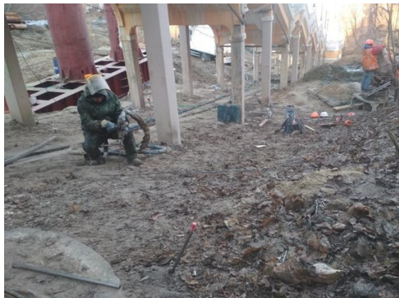
Fig. 16. The process of injecting polyurethane material into the soil under the foundations of the staircase supports at the construction site.
