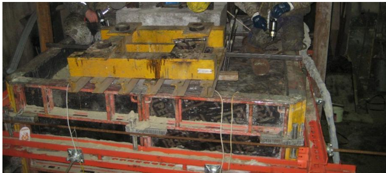
Fig. 12. Injection of polyurethane materials.
