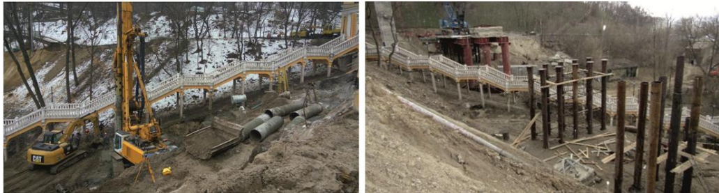
Fig. 7. View of temporary supports during their construction (2019).
