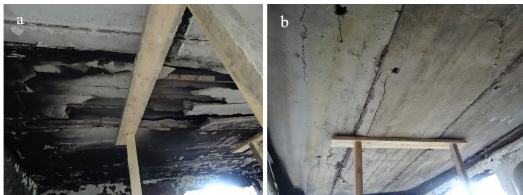
Fig. 4. General view of ceiling damaged by thermal impact: left – slab body falling out; right – lower zone cracking
