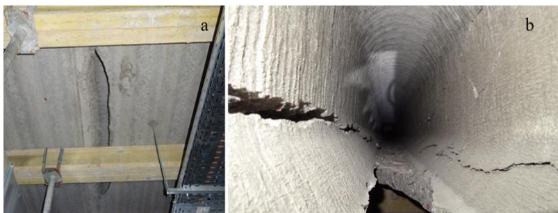
Fig. 14. Appearance of the damaged floor slab: left – bottom surface; right – interior space
