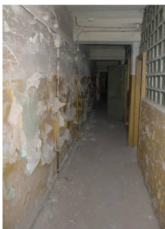
Fig. 10 Building B5 – dampness in the northern wall in the basement. Author of the picture: Dr. Eng. Jan Kozicki
