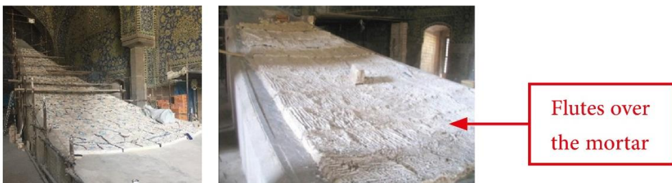
Fig. 25. Mortar pouring to the back of the Narreh mosaic over the curved mold and flutings of this somewhat denser mortar. Recent restoration of the Jame-Abbasi dome (source: CHO)
