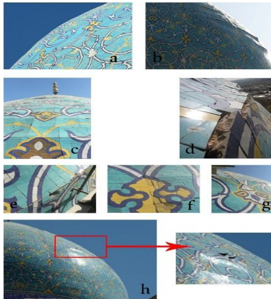
Fig. 3. Jame-Abbasi mosque dome: a. Inflamed tiles; b, h. Wrinkled tiles; c, d, e, g. Breaking and separation of tiles from the dome; f. Lack of adhesive mortar on the back of tiles after the 1980s and 1990s restorations
