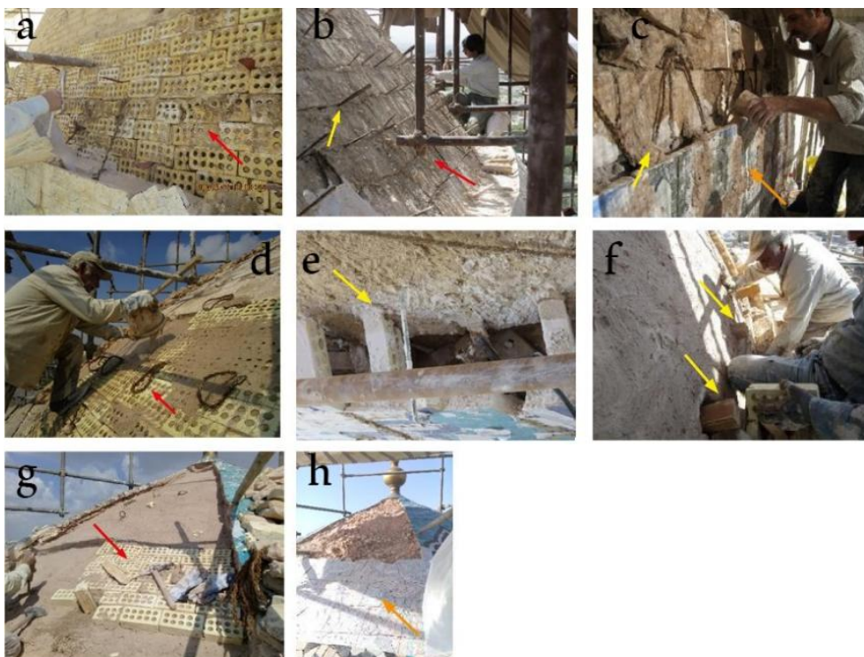
Fig. 28. Installation of hollow bricks (a, b, d, g; red arrow); installation of anthrax (b, f; yellow); installation of Parchehs of tile (c, h; orange); installation of Darab (c, e; yellow); gypsum mortar poured in back of the Parchehs (a, c, d; blue) (source: CHO)
