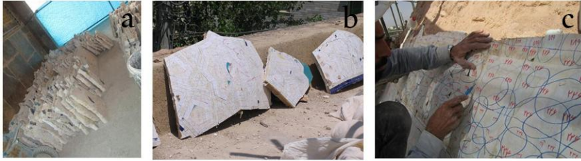
Fig. 22. Papers glued to the surface of the tile's Parcheh . a: Parchehs laid together in a recent restoration of the Jame-Abbasi dome to be installed on it; b: Parchehs of tile of another dome; c: Parchehs of tile in a recent restoration of Lotfollah mosque. (source: b. Enayati; a, c. CHO)
