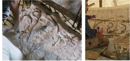
Fig. 14. Chaharbagh school dome, Gypsum mortar being poured on the back of Narreh tiles. (source: Panjehpoor)
