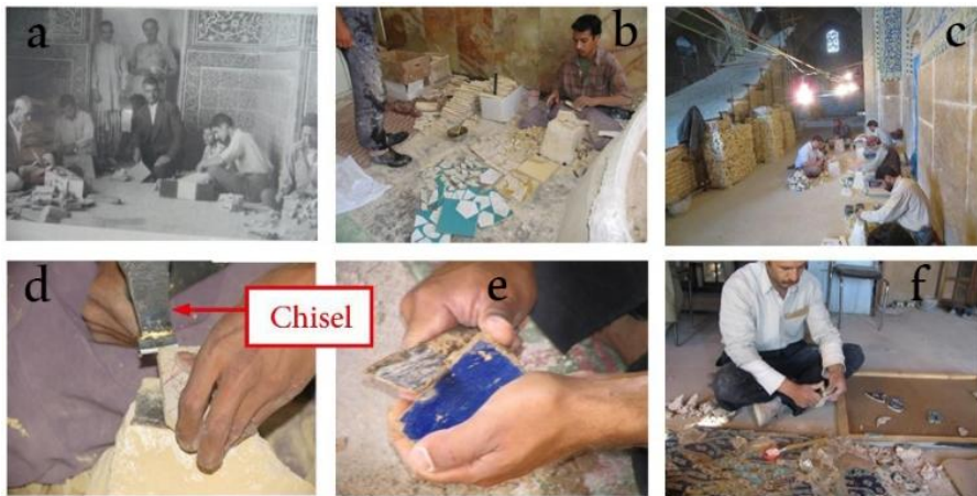
Fig. 23. a: Carving and chiseling of the tile in the past; b: Gluing of cut papers of the tile's design over the glazed surface of the tile by Sirish ; c: Chiseling and carving in a recent restoration workshop of Jame-Abbasi Mosque; d: Chiseling and carving; e, f: Removal of clay. (sources: top, CHO; bottom, Enayati)
