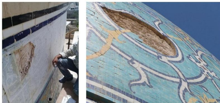
Fig. 31. Local restoration of dome's tiling (source: CHO)
