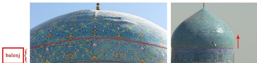
Fig. 2. Jame-Abbasi mosque dome, Balenj , or the impost of the dome: height determined by the arrow and the assumed horizontal line
