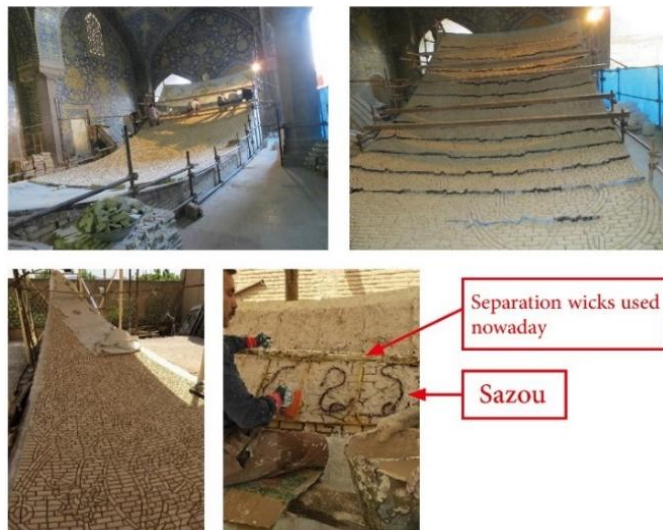
Fig. 24. Embedding of Narreh mosaic tiles inversely on the surface of the curved mold. (top): mold of Jame-Abbasi Mosque (source: CHO); (bottom): mold of dome, Chaharbagh school (source: Panjehpoor)
