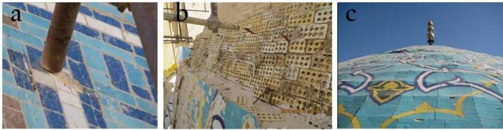
Fig. 32. a: Dome of Jame-Abbasi Mosque , damaged and broken tiles due to pressure exerted by buttress (Motalebi 2010); b: Dome of Chahar-bagh school , use of jackhammer to remove old mortar and its separation from tiling [39]; c: Dome of Jame-Abbasi Mosque , installation of anthraxs after that of tiles' Parchehs (Motalebi 2012)
