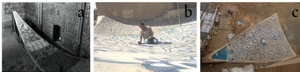
Fig. 21. a: Implementation of the design over the mold, using oils, of previous restorations of Jame-Abbasi Mosque ; b: Lotfollah Mosque , drawing of design over the mold of the dome; c: Lotfollah Mosque , completion of design over the curved mold. (source: a, b, c. CHO)
