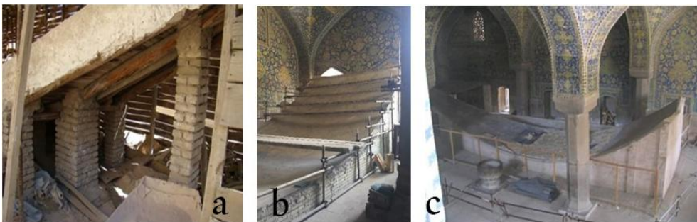
Fig. 19. a. the lower part of the old curved restoration mold of the Chahar-bagh school dome; b, c. curved mold of the recent restoration of the Jame-Abbasi Mosque tiling dome (sources: a. Motalebi 2010; b, c. CHO)
