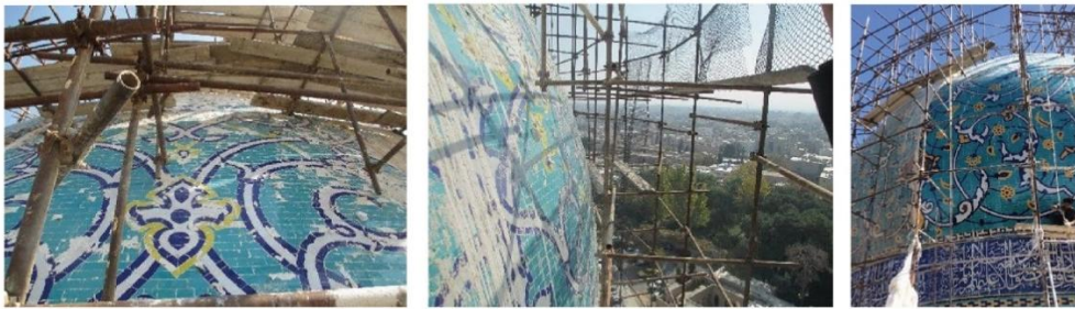
Fig. 30. Dome of Jame-Abbasi , after Dough-ab pouring and jointing, but before cleaning (source: CHO)
