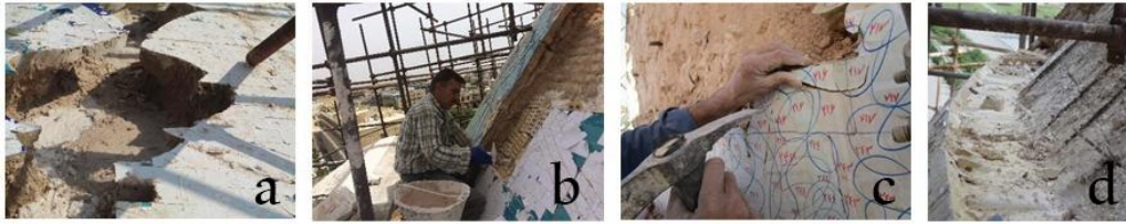
Fig. 29. a: Parchehs of tile involving a distension; b, c: modification and addition of some of the tiles after installation of Parchehs ; d: and after Dough-ab pouring (source: CHO)
