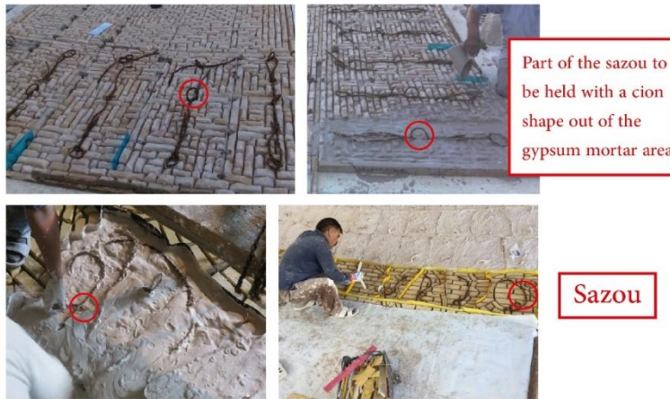
Fig. 26. Gypsum mortar with the Sazou rope at the back of the tile and the separating “walls” of each Parcheh ; (top): Lotfollah Mosque’s dome restoration (source: CHO); (bottom): Chahar-bagh school’s dome restoration (source: Panjehpoor)
