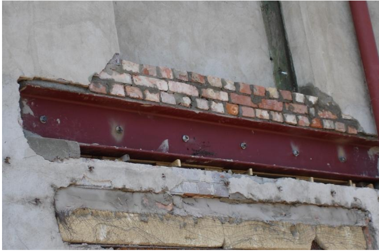
Fig. 7. New lintel (strengthening the structure in light of new utility requirements) at the location of the widened existing opening
