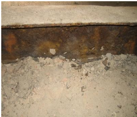
Fig. 5. Corrosion of existing ceiling beams
