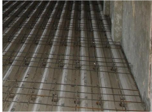
Fig. 4. New composite floor before pouring the slab
