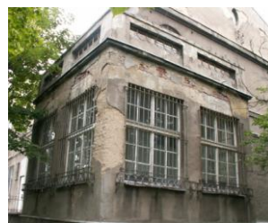
Fig. 3. Surface detachment of plaster within the first floor (author's photos: A. Kysiak)
