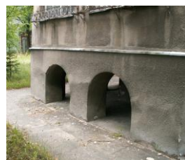
Fig. 6. Traces of plaster dampness in the plinth zone (author's photos: A. Kysiak)
