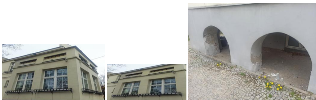
Fig. 29. Building elevation after renovation – visible original, restored window joinery and refurbished original flower grilles beneath the windows (author's photos: N.Solkiewicz-Kos, M.Tubielewicz-Michalczuk)
