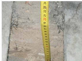
Fig. 11. Beam height measurement ceiling above the first floor (author's photos: A. Kysiak)
