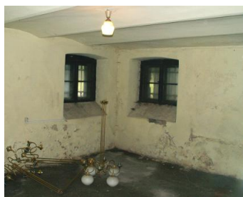
Fig. 7. Dampness of basement walls in the southwest. (author's photos: A. Kysiak)
