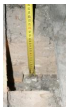
Fig. 11. Beam height measurement ceiling above the first floor (author's photos: A. Kysiak)
