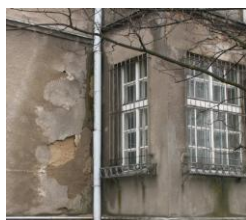
Fig. 5. Stains and dampness on the walls in the area of the leaking downpipe (author's photos: A. Kysiak)
