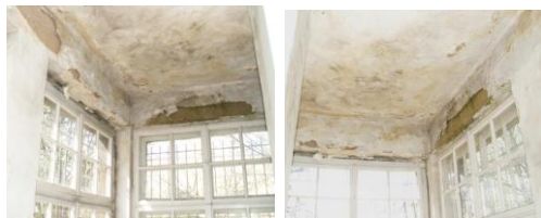
Fig. 10. Dampness, rotting plaster and brick, mold infestation of the walls in the veranda on the ground floor (author's photos: A. Kysiak)
