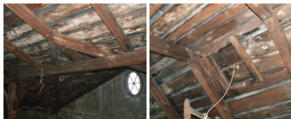
Fig. 15. Technical condition of the roof truss elements (author's photos: A. Kysiak)
