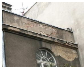
Fig. 4. Plaster loss and brick erosion at the ground floor level (author's photos: A. Kysiak)
