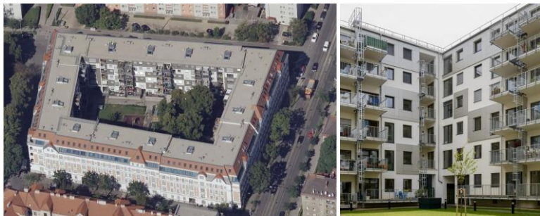
Fig. 4. An example pre-war housing tenements' renovation with balconies' additions, Lobmeyrhof in Ottakring, Vienna, Austria (source: Datenquelle: Stadt Wien – data.wien.gv.at https://www.wien.gv.at/stadtplan3d/#/ ) (left). Picture from courtyard perspective. Source: https://www.architektur-kiener.at/cms/2016/12/21/lobmeyrhof-1160-wien/ (right).
