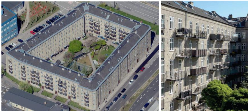
Fig. 3. An example of add-on cantilevered balconies to the elevation of pre-war tenement houses situated in quarters, Nørrebro district in Copenhagen, Danmark (source: https://skraafoto.dataforsyningen.dk/ ) (left). Picture from courtyard perspective. By: Nanna Nielsen, source: Stender 2021 (right).
