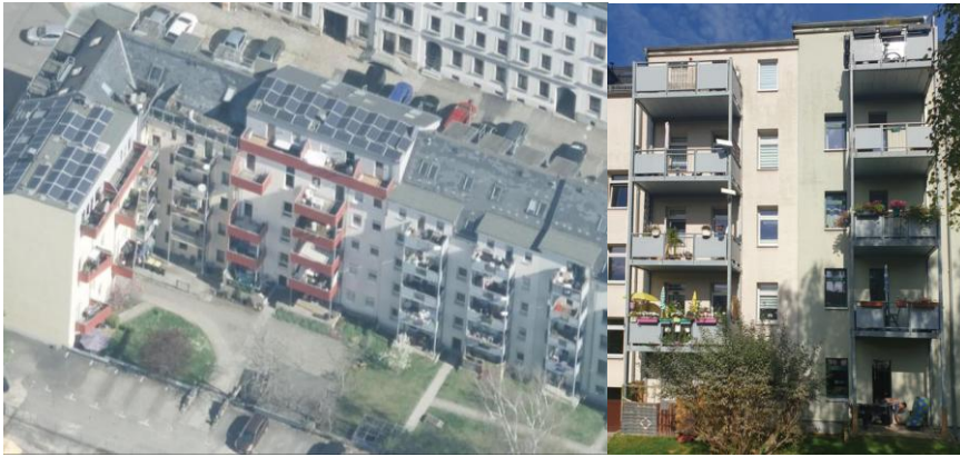
Fig. 2. An example of add-on balconies to the backyard elevation of tenement houses situated in quarters, Karl-Liebknecht-Street, Chemnitz, Germany (source: Data license Germany – attribution – version 2.0 https://www.govdata.de/dl-de/by-2-0 Städtisches Vermessungsamt Chemnitz https://chemnitz.maps.arcgis.com/ ) (left). Balcony additions at backyard elevation. Picture taken in presented courtyard during the fieldwork (right).
