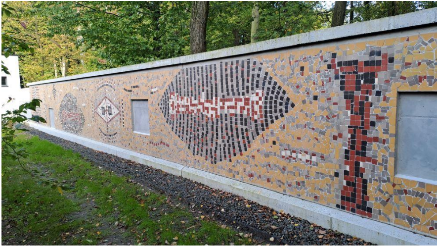
Fig. 24. Cracow Zoo—view of completed wall with mosaics exhibition
