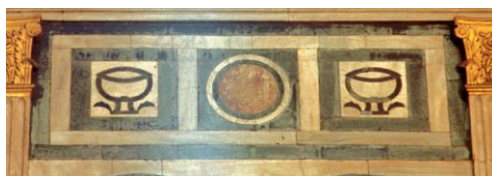
Fig. 24. Marble inlay above the central mullioned window on the southwest side ( second internal order or women's galleries )
