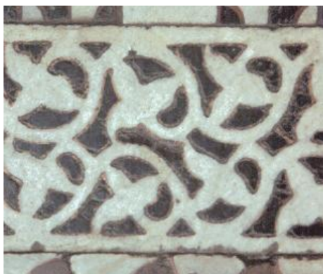
Fig. 6. Contour band of the baptistery flooring, featuring geometric decoration with girali (northeast sector)
