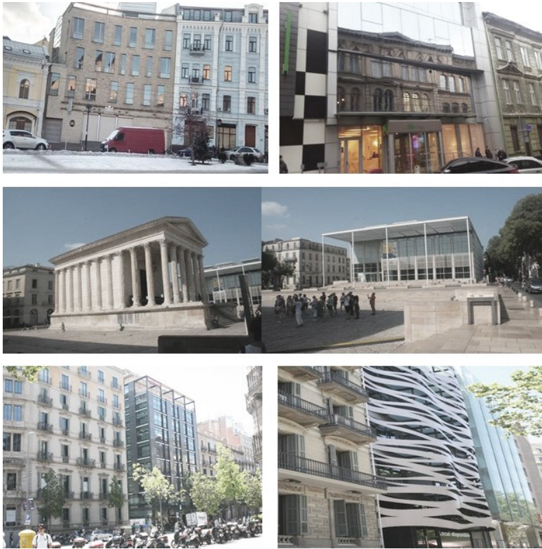
Fig. 4. Modern methods of new construction in a historical environment. The upper row (from the left) is the building of the Embassy of the Netherlands in Kyiv (arch. Hans van Beek, D. Zaplatnikov, A. Khmelov); on the right, the facade of the Ibis hotel, which mirrors the facades of the slums of the opposite side of the street; in the middle – the Saree Art Center in Nîmes, France (arch. Norman Foster) – a building with glass facades, which is also a paraphrase of a monument of the ancient era; the bottom row of the newest houses in the architecture of the new streets of Barcelona.
