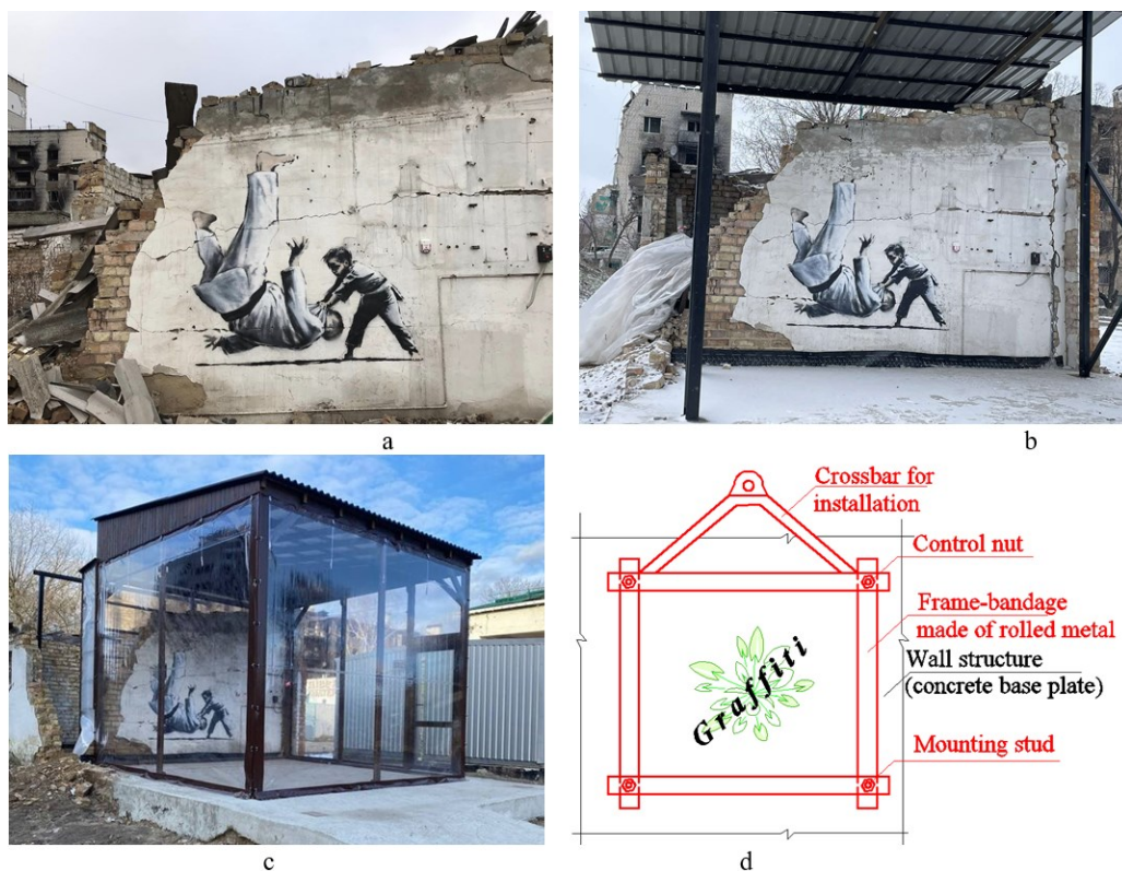
Fig. 9. Protective structure over the graffiti «Judoists» in Borodyanka: a - november 2022; b - february 2023; c - march 2023; d - schematic diagram of a frame-bandage for a fragment of a wall – front view.
