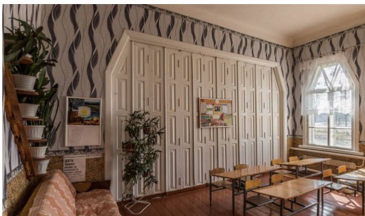
Fig. 6. Sliding door between classrooms in the school of the village Mlyny Lokhvytsia district (1911)
