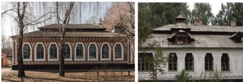
Fig. 8. Pitched roof with characteristic folds and windows preserved in schools in the villages of Haivshchyna (on the left) and Bodakva (on the right)
