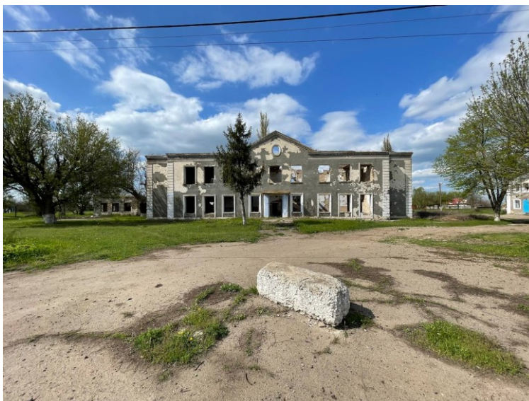
Fig. 10. Demolished building in Mikolayev region [Photo by Serhii Belinskyi, 2022]
