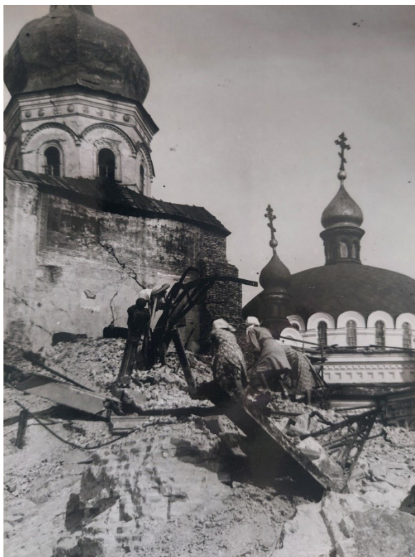
Fig. 9. Demolition of the ruins of the Cathedral of the Assumption [Photo: Archive Ukrrestauratsiya Corporation]
