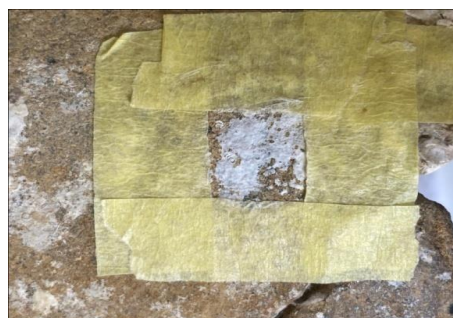
Fig.11. Result of citric acid cleaning
