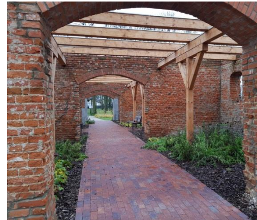
Fig. 12. The roof of the former barn was changed into a pergola. Currently, the building serves as a garden-art gallery
