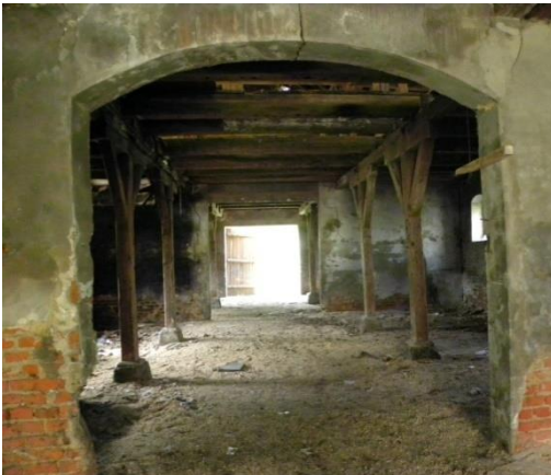
Fig. 11. View of the ruins of the former cowshed
