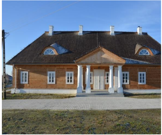
Fig. 18. The manor house after renovation, 2020
