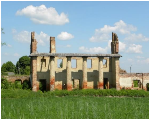
Fig. 7. View of the ruins of the orangery in Zawieprzyce
