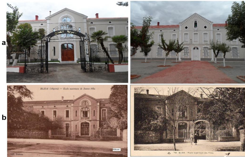
Fig. 3. El Feth High School between the past and the present: a - El Feth High School in the present. Source: Design office Bouras; b - El Feth High School in the past. Source: www.Blida.net
