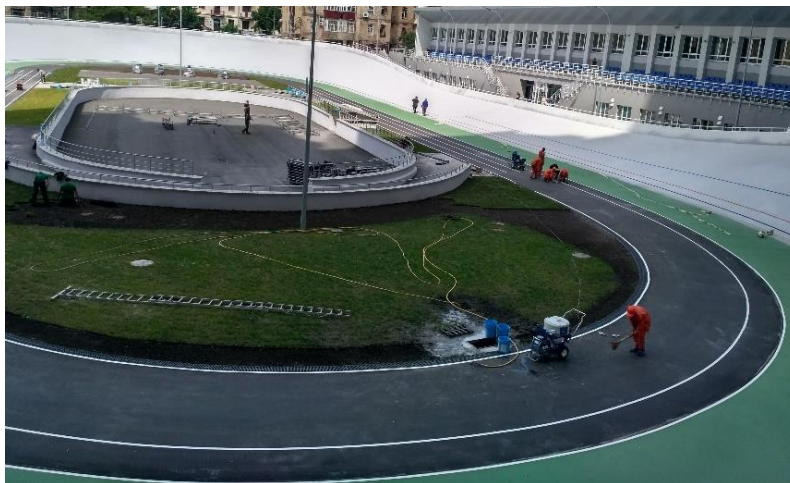
Fig. 14. The Kyiv is in the final stage of work.
