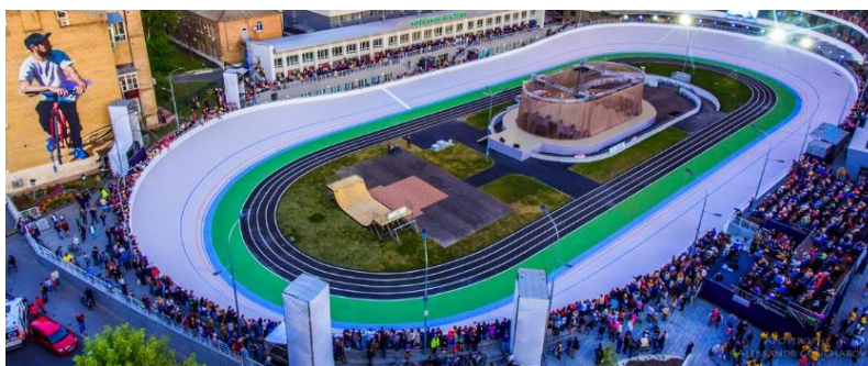
Fig. 5. View of Kyiv Velodrome after restoration in 2017. [Source: https://apostrophe.ua/ ]
