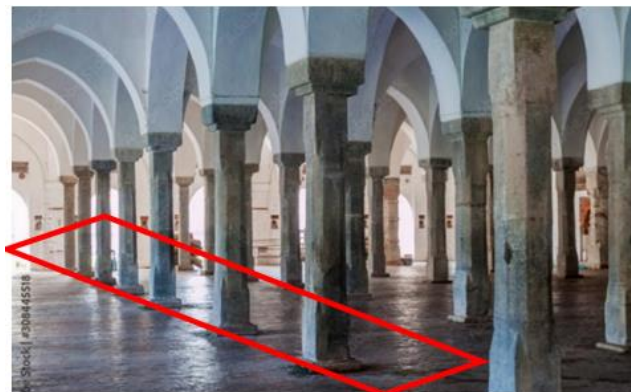
Fig. 7. 4” pillar-base to protect them from dampness
