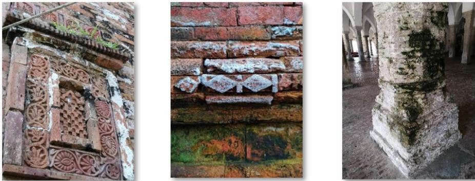
Fig. 10. Crystal formation of salt and erosion of the building materials in Khalifatabad
