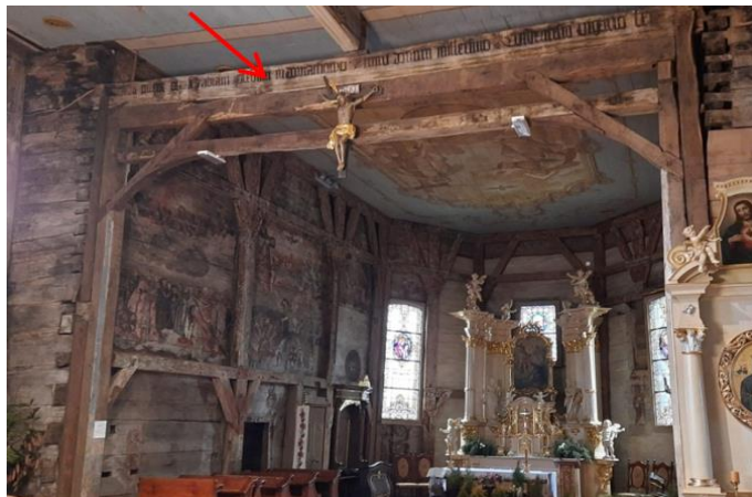
Fig. 3. View of the rood beam from the nave side
