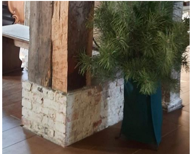
Fig. 23. A multi-branched column set on a brick plinth
