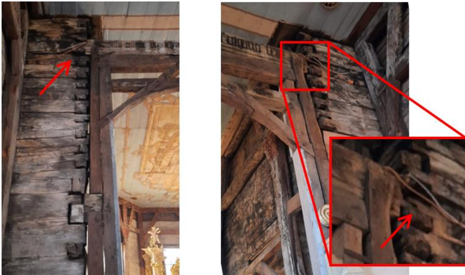
Fig. 19. Fragments of short log walls at the junction between the nave and chancel
