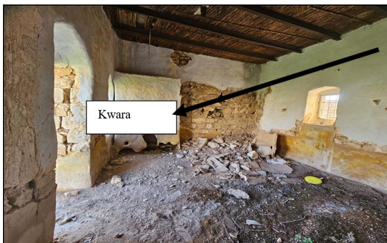
Fig. 10. Showing the clay floor of the house and the front of the photo is a wheat storage called Kwara
