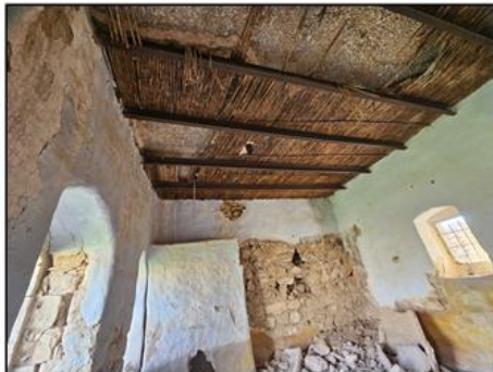
Fig. 9. Showing iron bridge carrying the sugarcane wood beams and another component in the roof: a. showing wooden bridge carrying sugarcane wood on Arch-shaped structure; b. Iron bridge caring sugarcane beam on a regular flat roof
