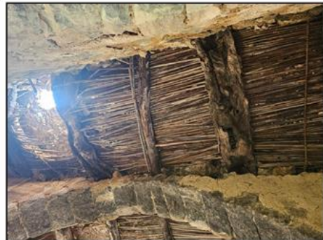
Fig. 9. Showing iron bridge carrying the sugarcane wood beams and another component in the roof: a. showing wooden bridge carrying sugarcane wood on Arch-shaped structure; b. Iron bridge caring sugarcane beam on a regular flat roof
