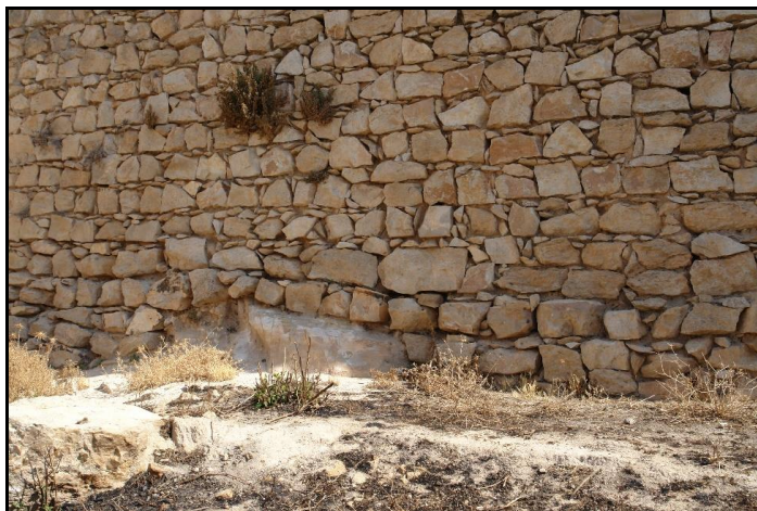
Fig. 6. Shows the elastration rows of stones and their reinforcement with small stone on continuous bedrock
