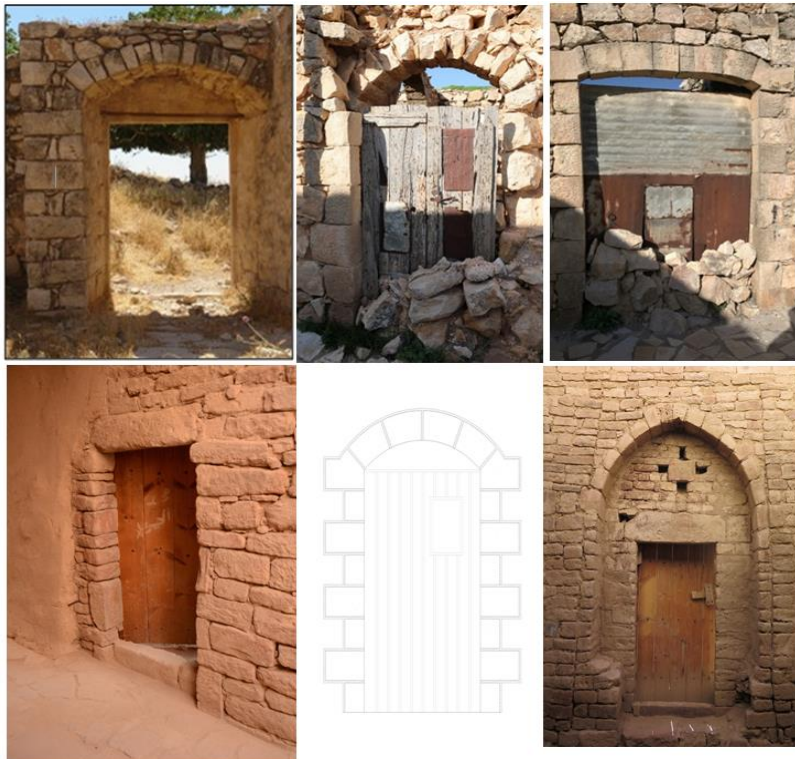
Fig. 12. A collection of door patterns in the village showing how the arches are built and the doors are made of wood and iron
