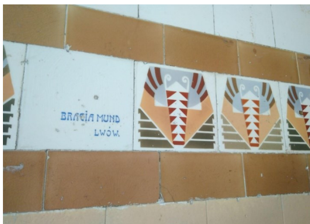
Fig. 4. Ceramic facing tiles in the decoration of walls in the entrance space of a residential building located at 31 Volynska Street, Lviv.
