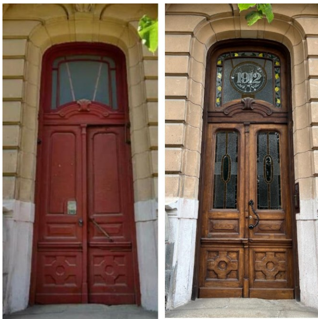
Fig. 1. Entrance doors in a residential building located at 1 Korolya Danyla Street, Ivano-Frankivsk (before and after restoration).
