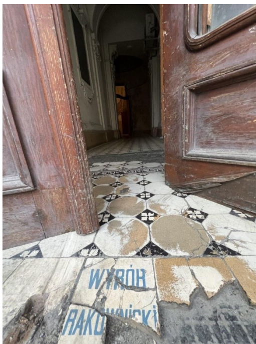
Fig. 3. Ceramic Mettlach tile in the entrance space of a residential building located at 8 Acad. V. Hnatiuka Street, Lviv.
