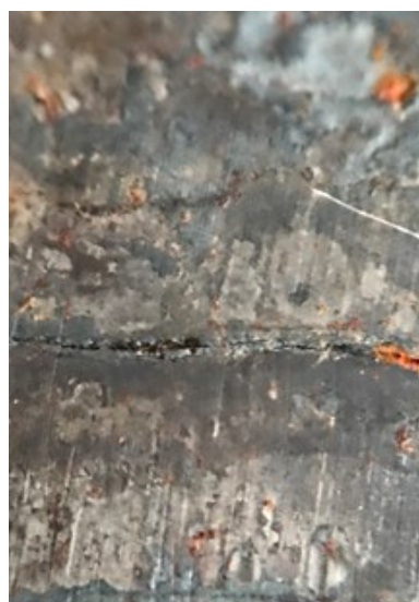
Fig. 9. Visible crack in the material
